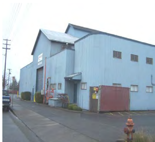
Painted Siding and Roof
