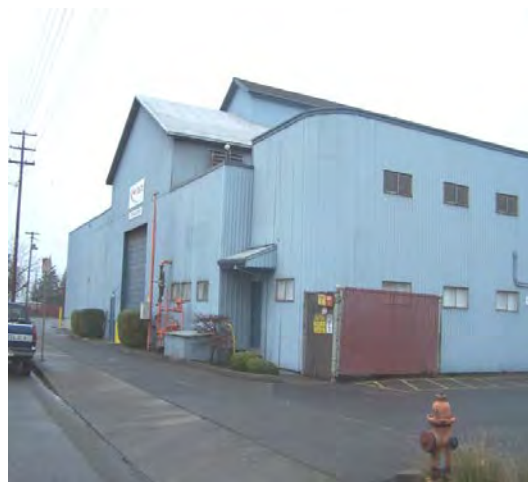
Painted Siding and Roof
