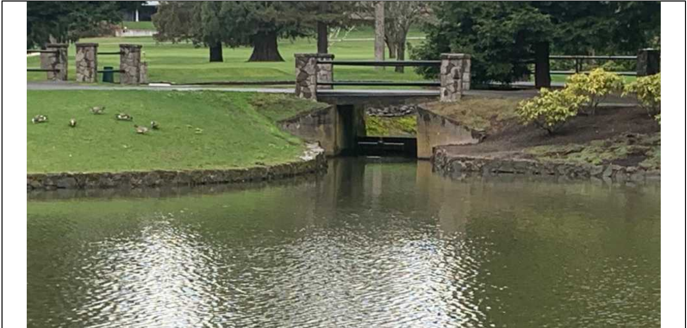
View northwest at water control gate between irrigation pond and Fanno Creek. View of upgradient side of water control gate, which detains water from Woods Creek.
