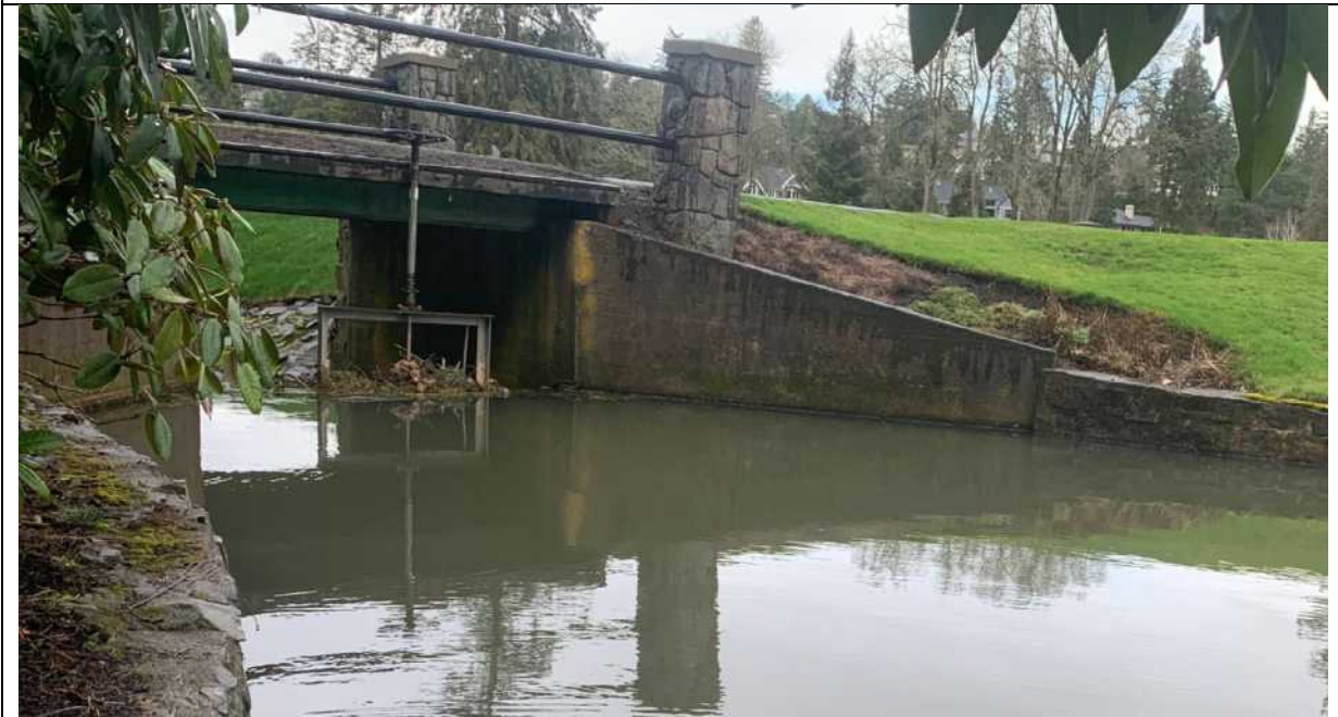
View northwest at water control gate that impounds Woods Creek and detains water for irrigation pond. View of upgradient side of water control gate.
