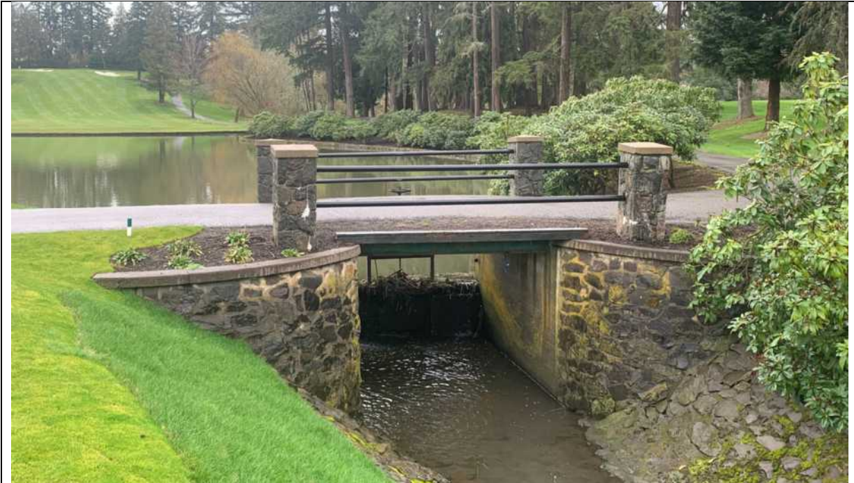
View east at water control gate that impounds Woods Creek and detains water for irrigation pond. View of downgradient side of water control gate.
