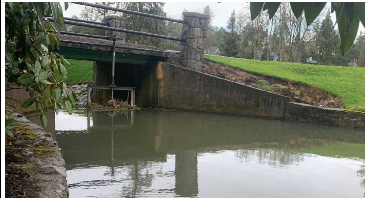
View northwest at water control gate that impounds Woods Creek and detains water for irrigation pond. View of upgradient side of water control gate.
