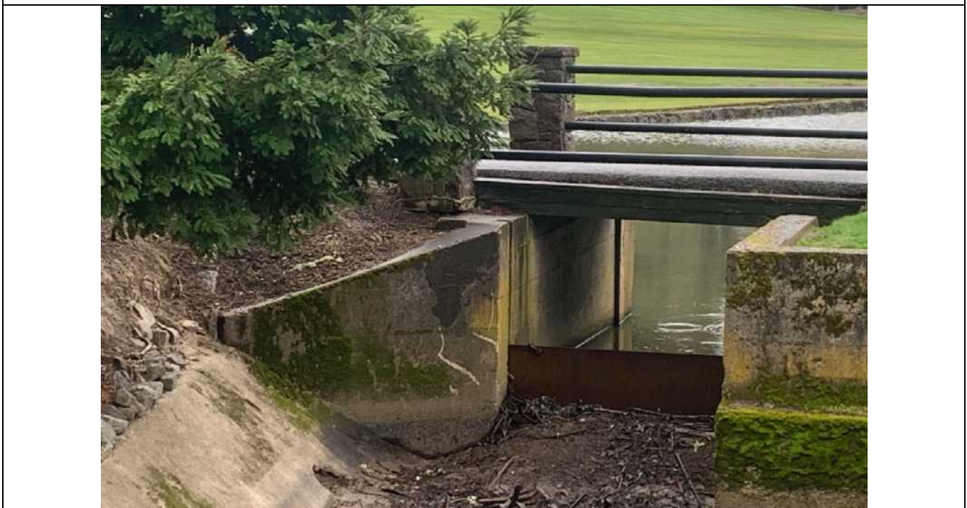
View southeast at water control gate between irrigation pond and Fanno Creek. View of downgradient side of water control gate. Floating debris from Fanno Creek is stopped from entering irrigation pond.
